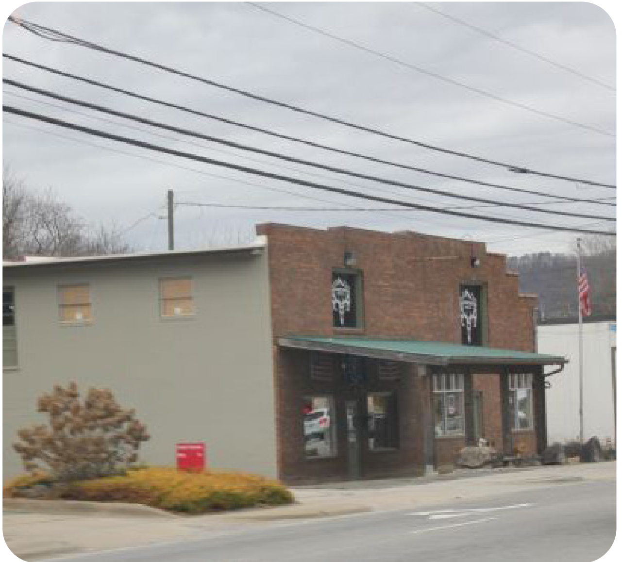
Tagged Out hunting supply is able to keep their location but anticipates losing several feet off of the front of their business. Photo by WCJ.
